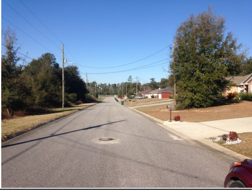
Street View – West
